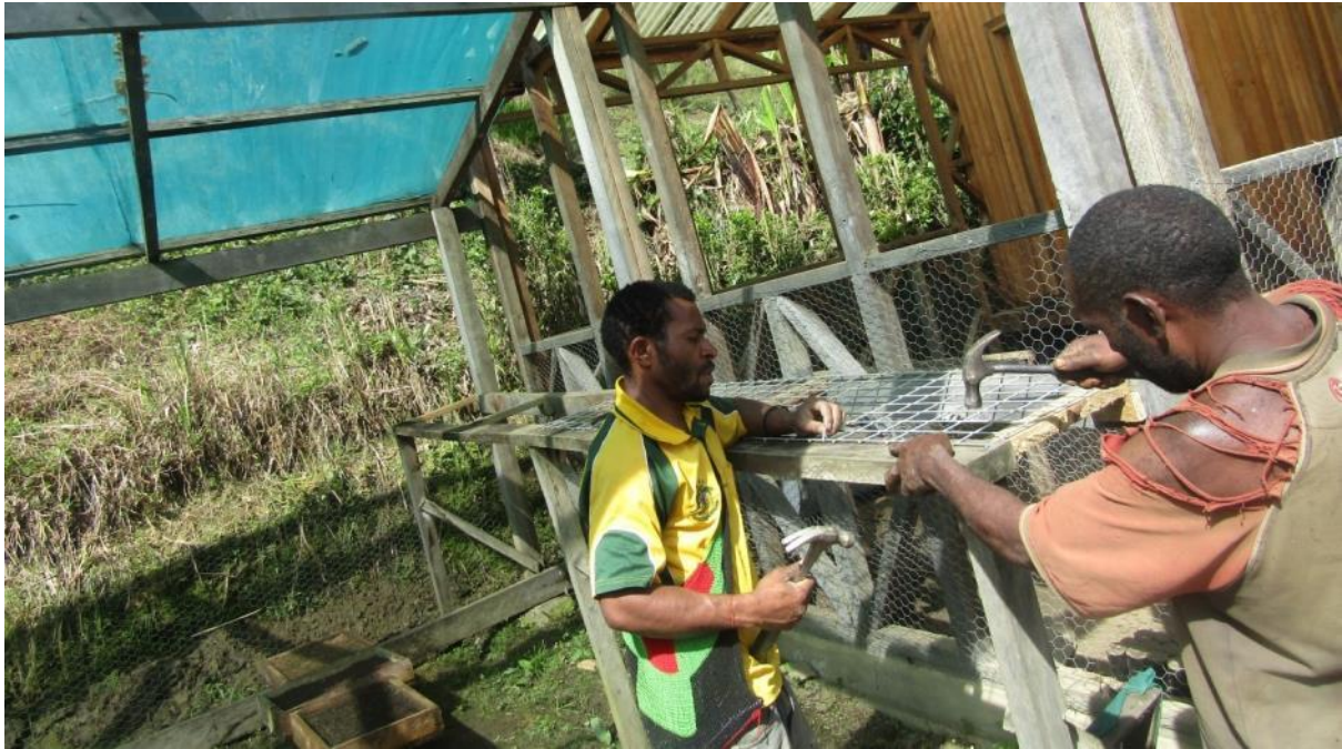
Figure 7: Shelf repair for installation of germination trays (KGWan Eco-habitat nursery - Danbagl)
